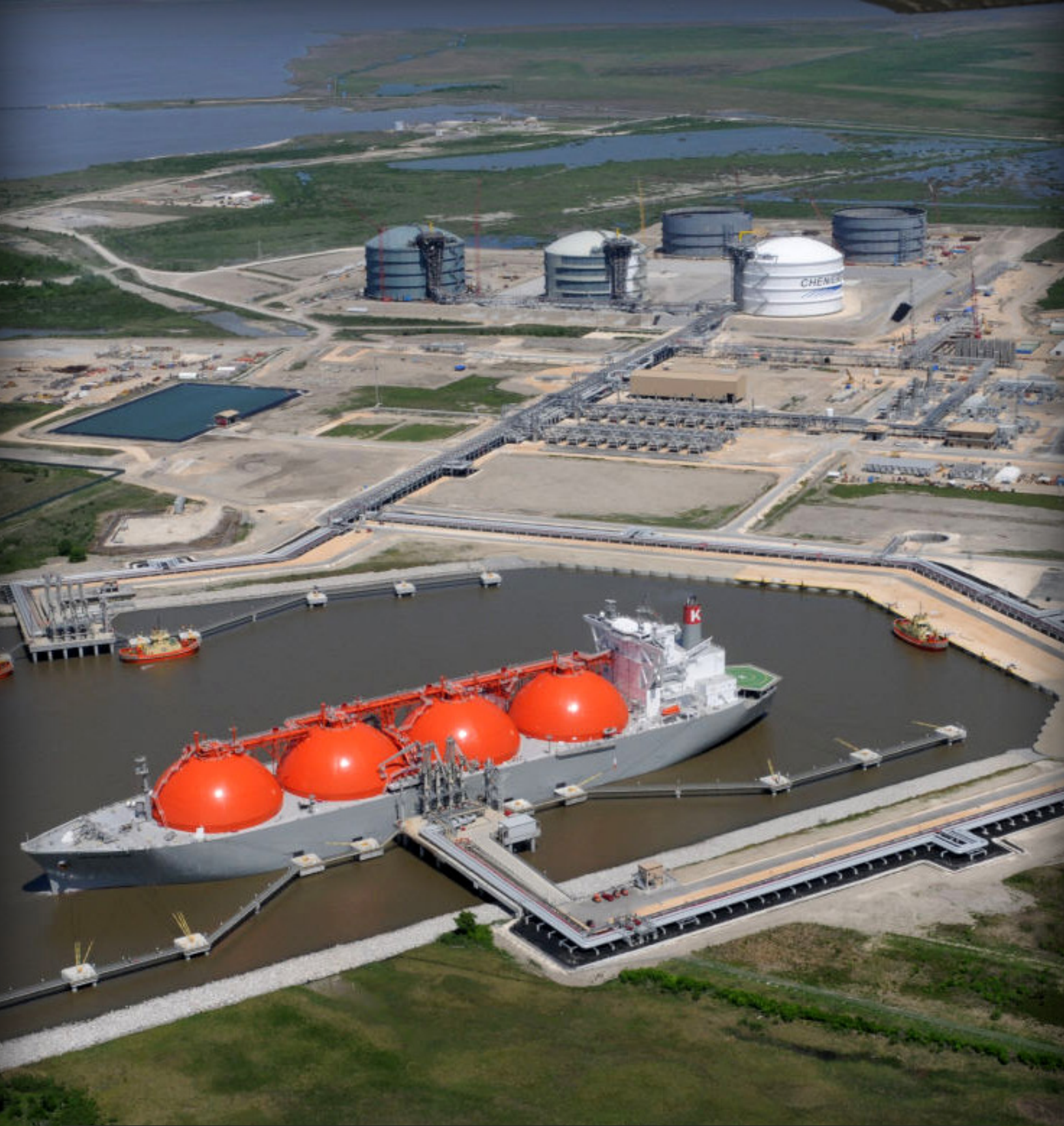
An aerial shot of the Sabine Pass LNG Terminal in Cameron Parish, Louisiana. Operated since 2008, the terminal is now undergoing renovations to add gas liquefaction services. (Flickr user "Think Defense", CC license BY-NC 2.0)
